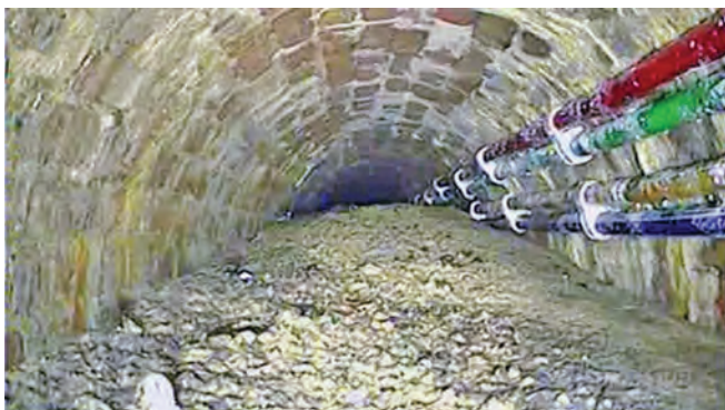
Concreteberg at the junction of Goswell Road and Hall Street, Islington
